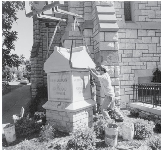
In fall 2000, workers lowered a 4,000-pound limestone capstone on a new sign for St. Margaret of Scotland as part of its centennial celebration.
